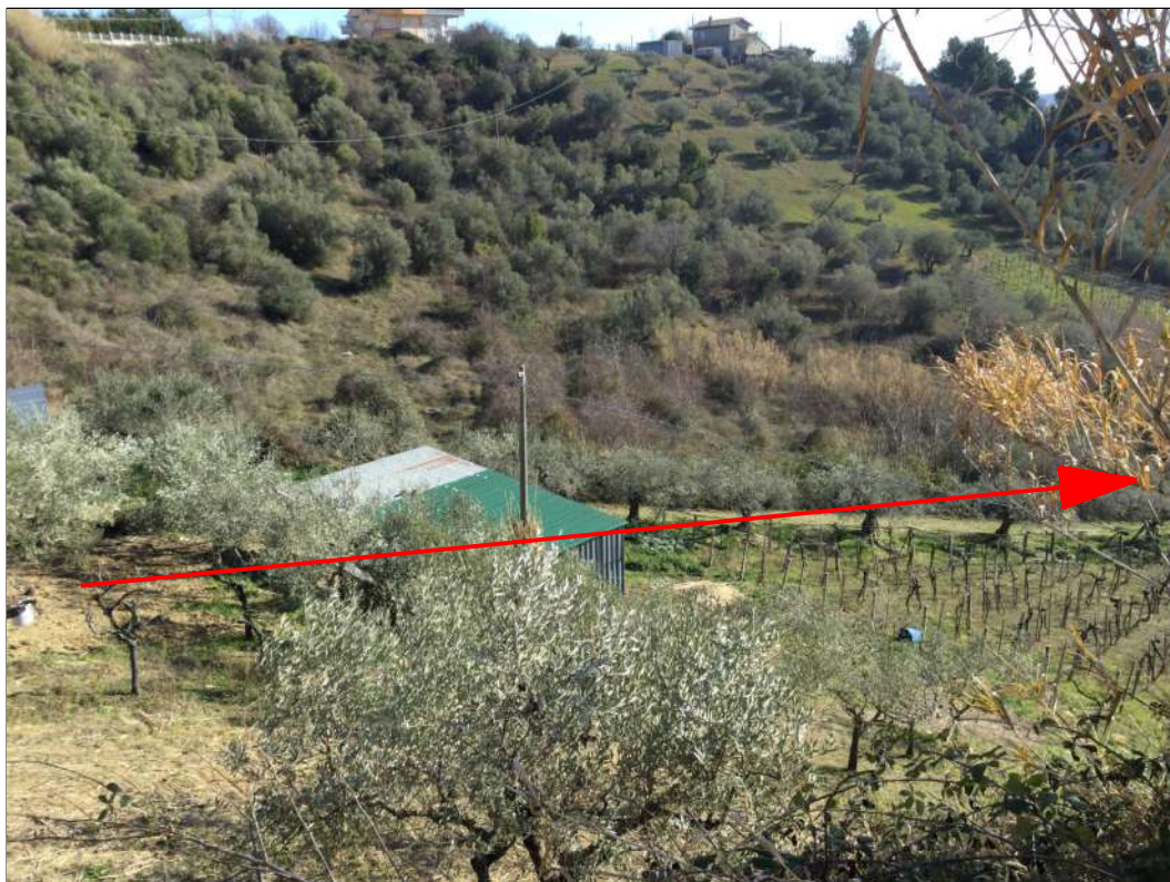
Trenchless (TOC Valle Furci)
